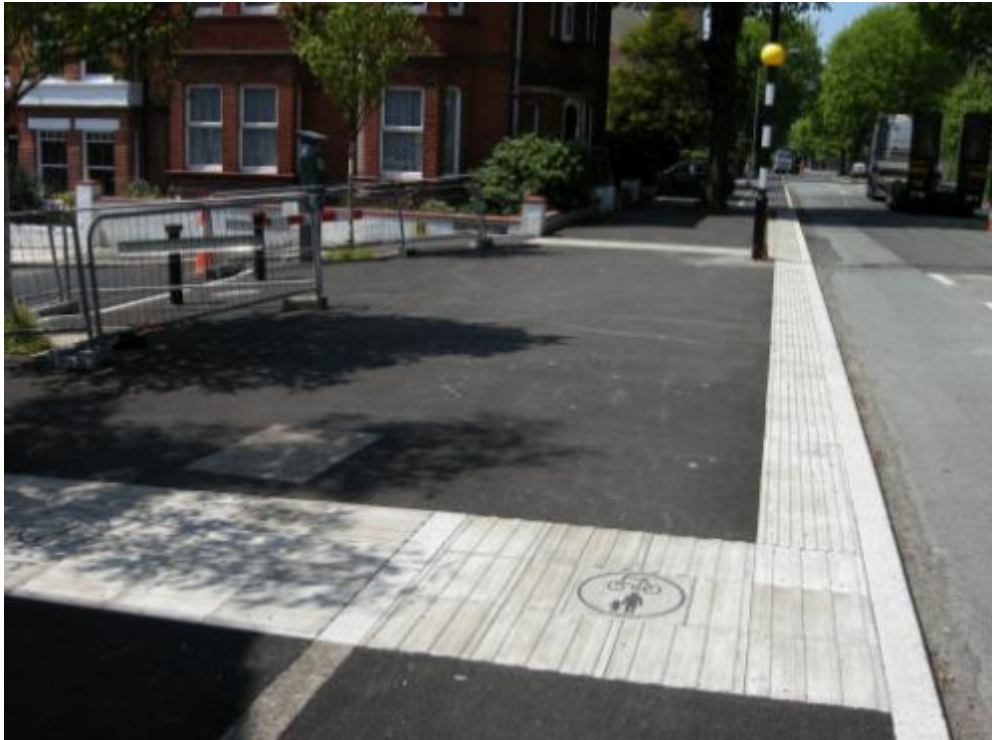
Filtered permeability where a residential side road meets a cycle track on a main road (under construction on Old Shoreham Road, Brighton). Not only does this arrangement remove rat-running on the residential street, it also eliminates turning conflicts across the cycle track.
